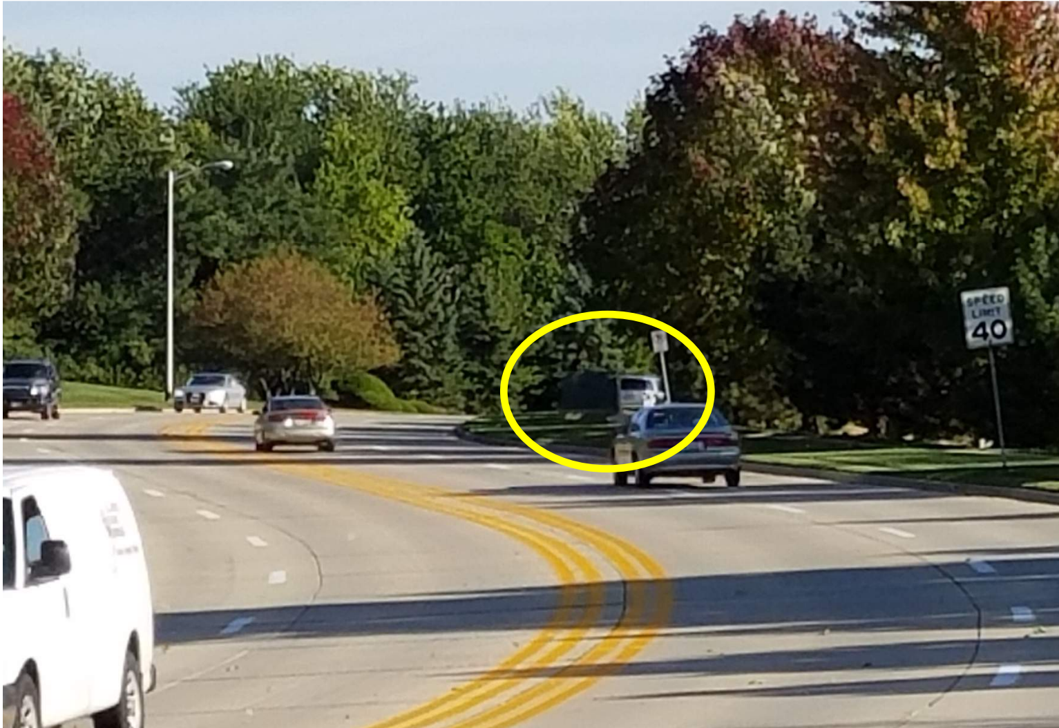
Photo 11: Looking Right to 897 feet (MU @ 50 mph) Visible Gap Between Utility Cabinet and Trees Illustrated by Vehicle
