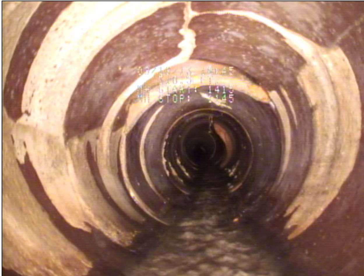
Clayton Street Sewer: Hinge cracking in clay sewer
