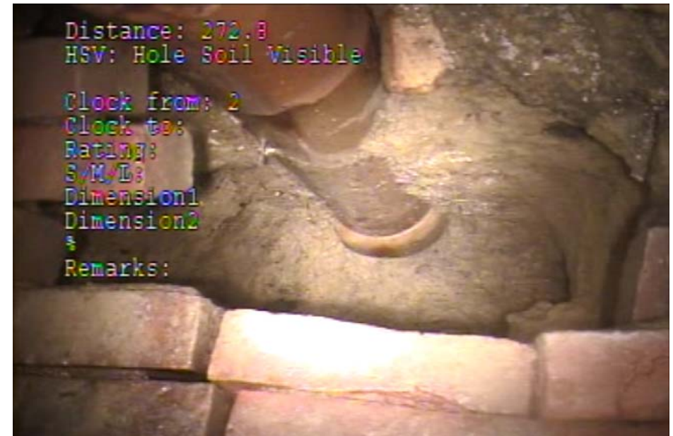
Holes in the Douglas Street Sewers filmed by CCTV
