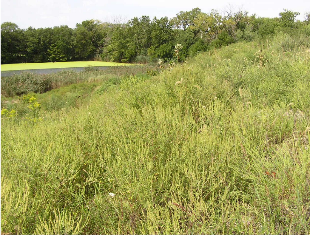
Date:09-04-2014 Time: 12:45PM Direction: Northwest Photo by: Jen O'Hearn Exposure #: 015 Comments: View along edge of excavation.
