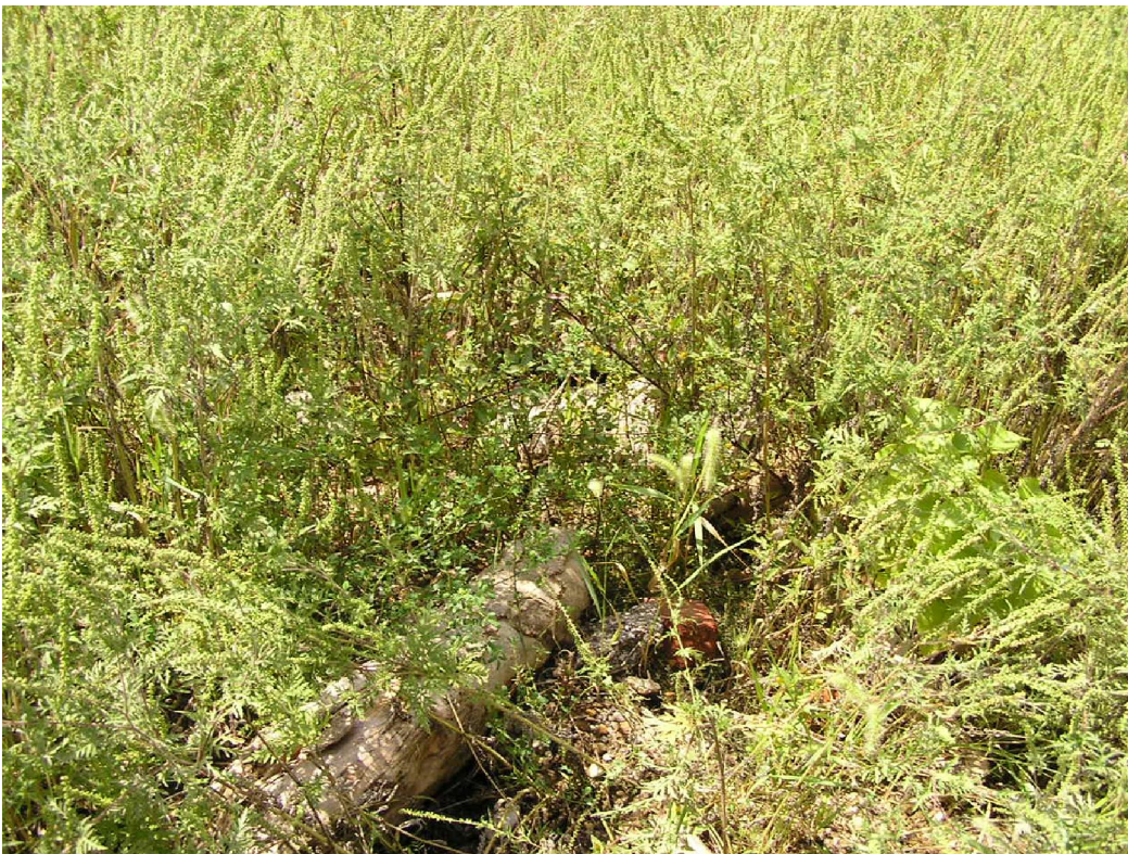
Date:09-04-2014 Time: 12:48PM Direction: Southwest Photo by: Jen O'Hearn Exposure #: 016 Comments: View of brick and asphalt on slope of excavation.
