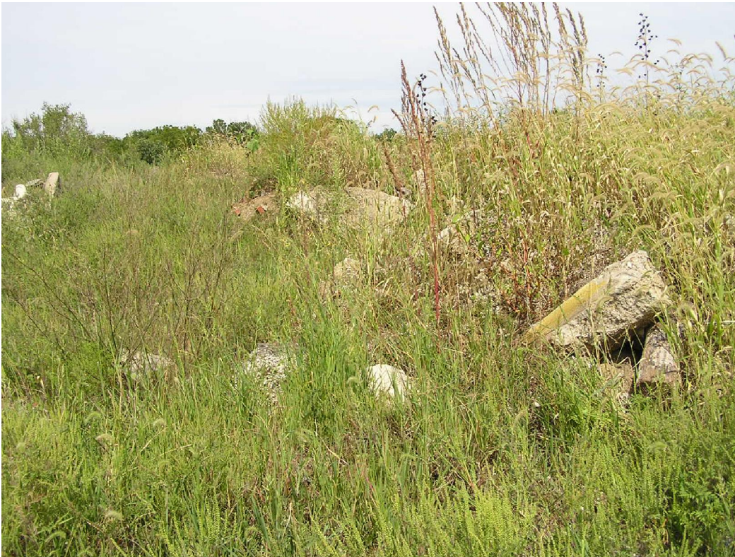
Date:09-04-2014 Time: 12:45PM Direction: Northwest Photo by: Jen O'Hearn Exposure #: 013 Comments: View of one apparent painted curb piece of concrete and concrete pieces in the weeds.
