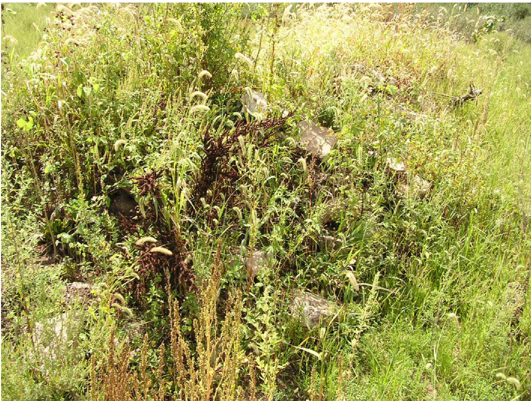
Date:09-04-2014 Time: 12:41PM Direction: Southwest Photo by: Jen O'Hearn Exposure #: 010 Comments: View of concrete in with soil pile with weeds growing.
