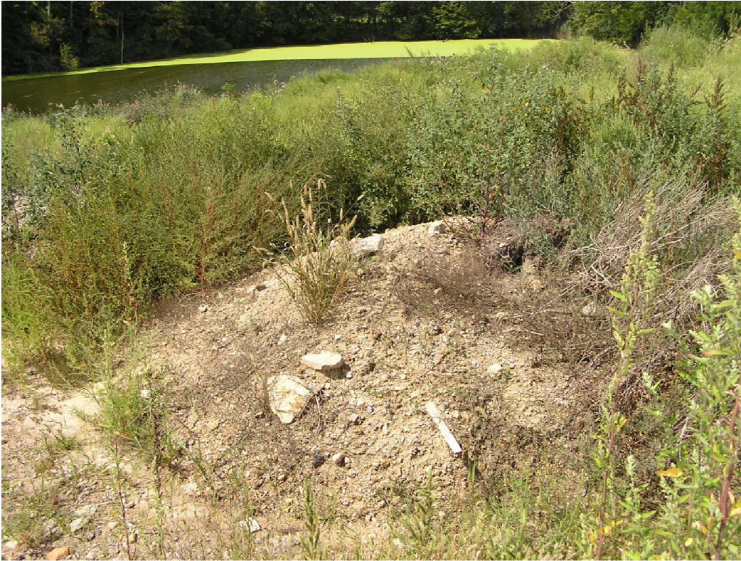
Date:09-04-2014 Time: 1:01PM Direction: Southwest Photo by: Jen O'Hearn Exposure #: 023 Comments: View of surveyor's stake and concrete in soil pile.
