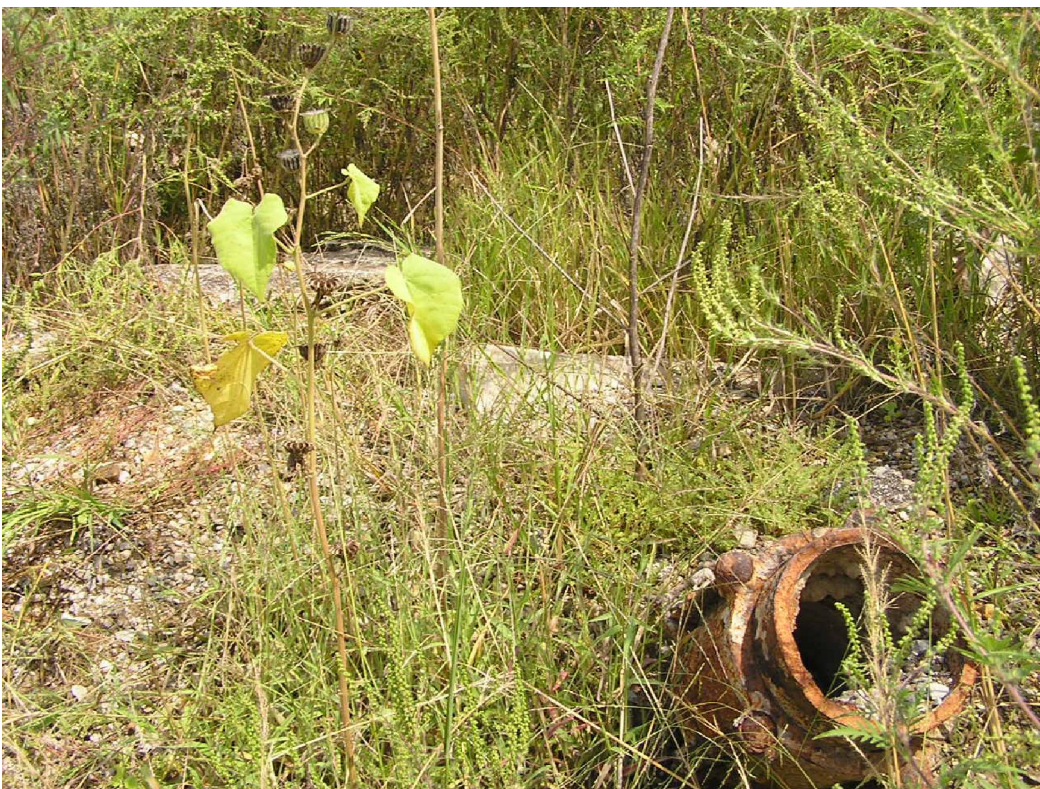
Date:09-04-2014 Time: 12:50PM Direction: Northeast Photo by: Jen O'Hearn Exposure #: 018 Comments: View of metal pipe looking up slope of excavation.
