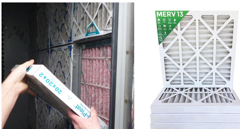
Figure 5: Pre-filter (MERV8) & final filter (MERV13) vs. Pre-filter (MERV13)
